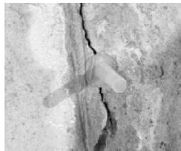
2. Remove the cap from the surface port, then apply a small amount of mixed adhesive to the bottom of the port base. Place the first port starting at the bottom of the crack and repeat every 8 inches until the
