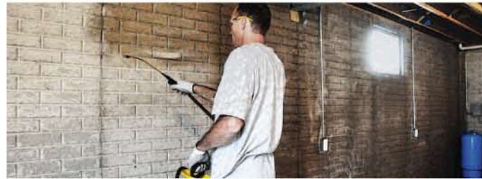
Saturate the surface by spraying on a continuous wetting film.
