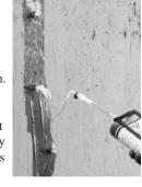
Hint: To improve the ability to penetrate very small & hairline cracks, heat the injection urethane system by placing the injection cartridge in a pail of hot tap water for 15-20 minutes. This temperature exposure should thin the material so that it can flow into the crack with less resistance proceed as before.
