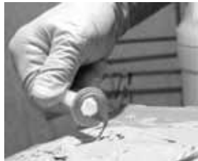
Adhesive applied to bottom of port base
