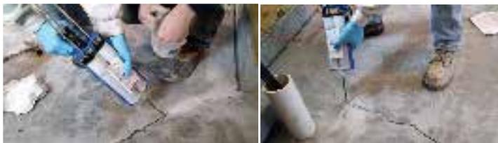
**TIP** - Maintain a steady flow of CrackWeld through the mixing nozzle or it may become plugged after a couple of minutes. After a stoppage, purge the mixer into a disposable cup. To minimize stoppages, repair small sections of the crack at a time (5-10 ft. or use up the whole cartridge).
