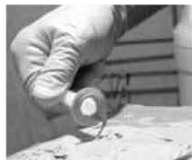
Adhesive applied to bottom of port base
