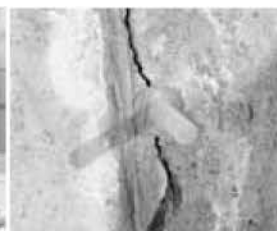
Center port over crack
